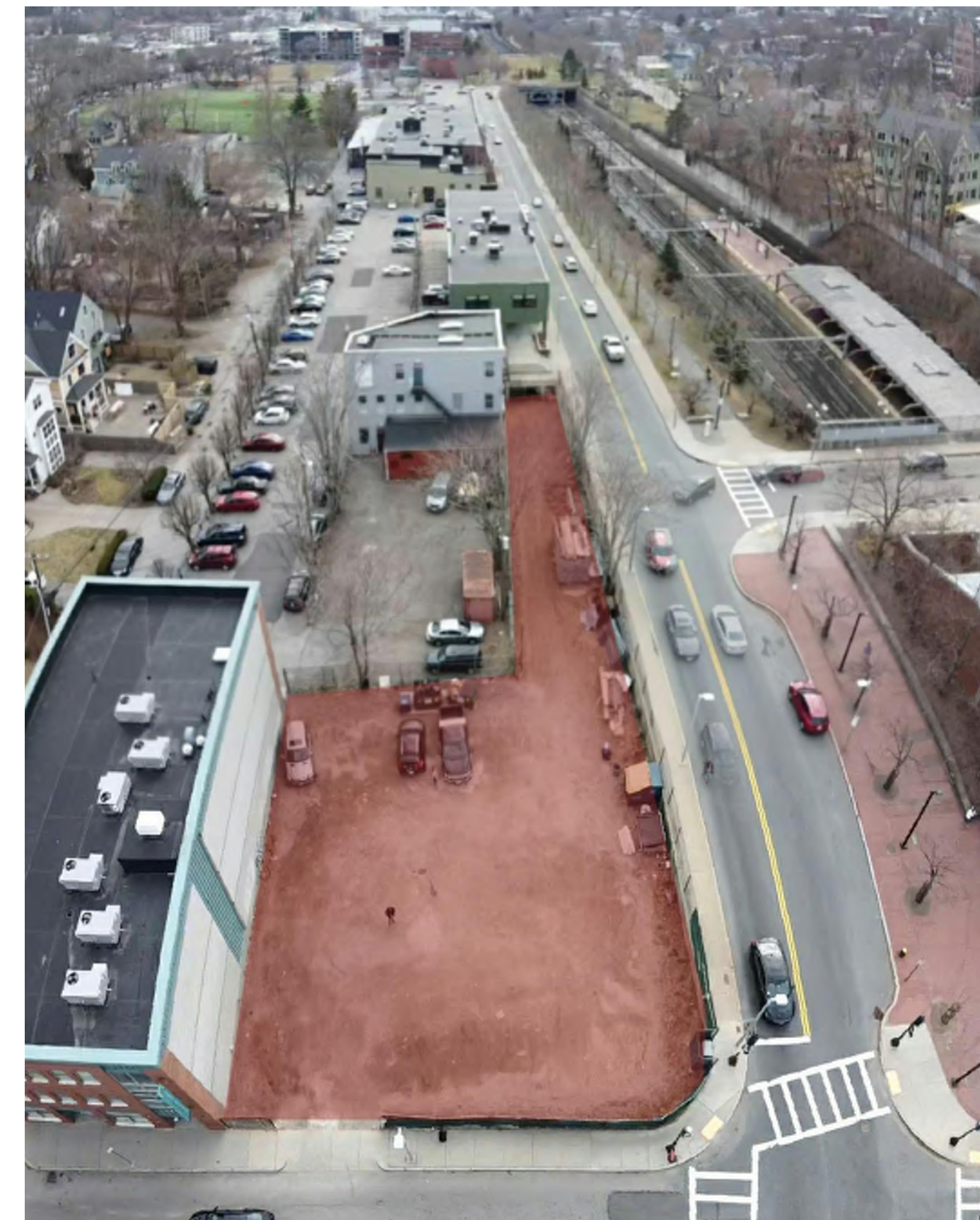
AERIAL VIEW OF EXISTING SITE
